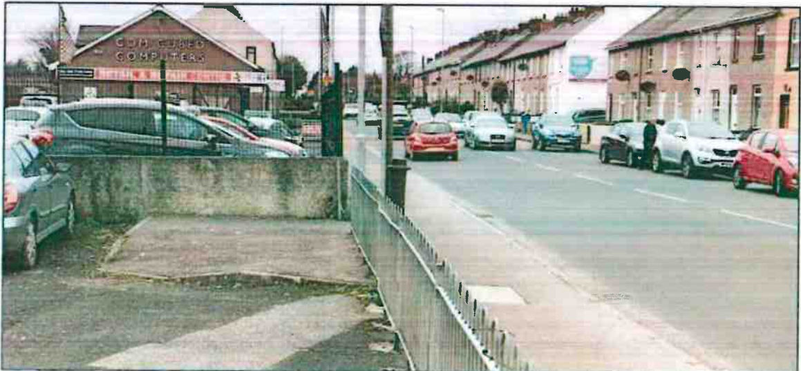
Photographs 2.1, 2.2 and 2.3: Views of the proposed site from the north eastern boundary
